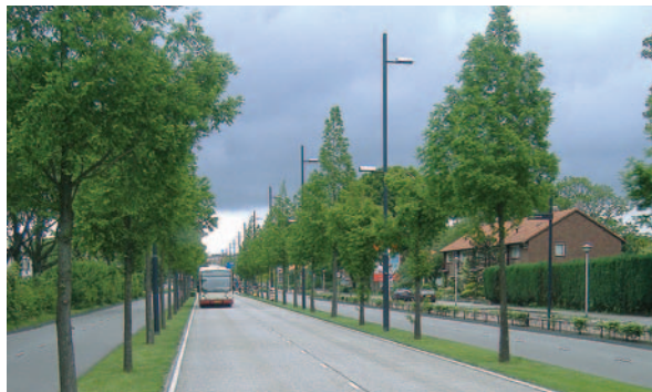
New-style Bus-way with new lighting columns interspersed with trees.
