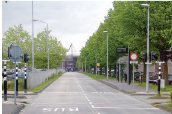
The Bus-way with dated lighting columns.
